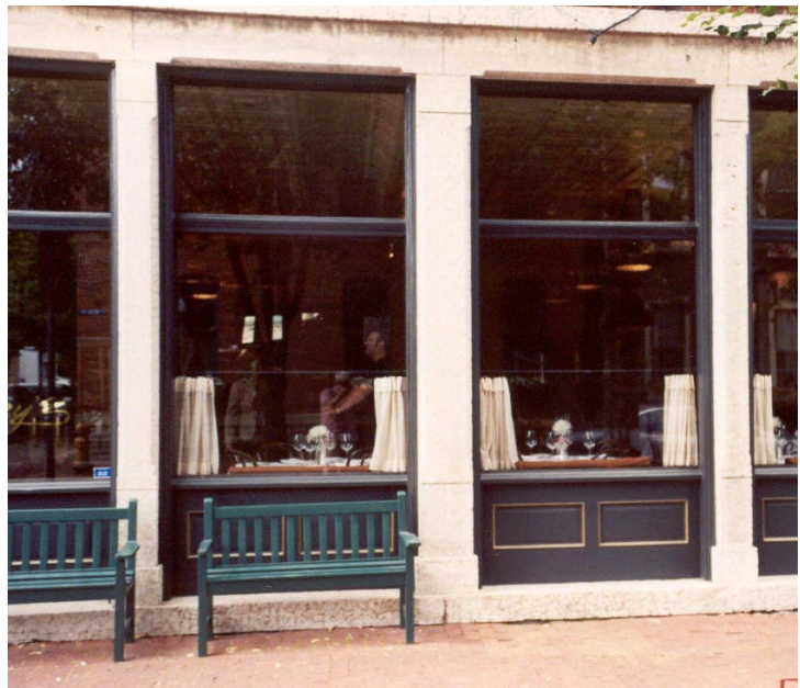
Storefront display windows typically had large panes of glass rather than smaller divided light glazing found in residential designs.
