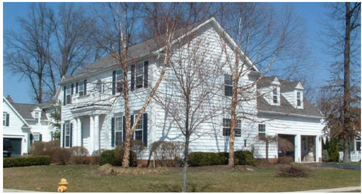
This building is oriented toward the street, with the wing containing a side-load garage secondary in character to the house
