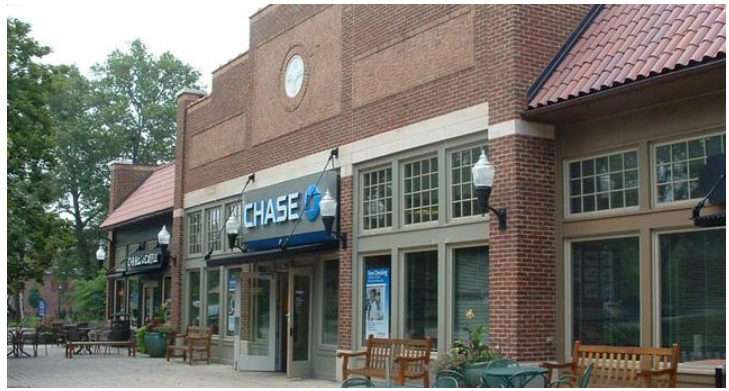
Commercial retail buildings outside the Village Center should avoid blank walls and create some pedestrian-friendly amenities.
