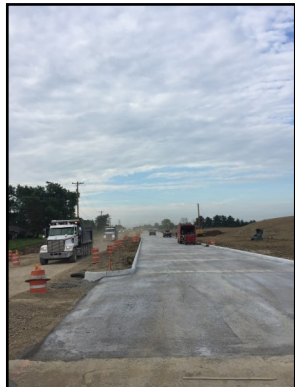
Beech Road Grading
