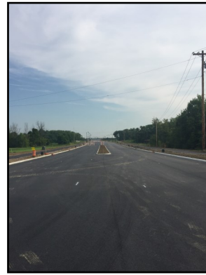
Northbound Beech Road
