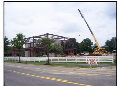
Walton Offices II
