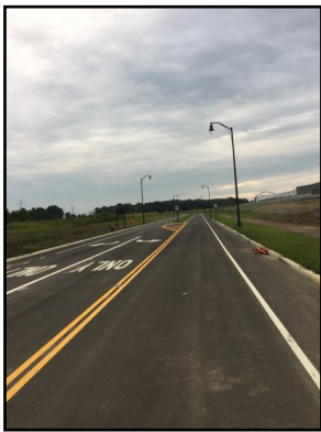
Loop Rd. Intersection
