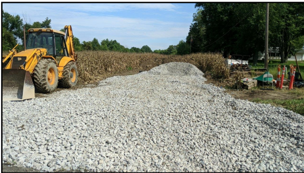
NAPD Morse Road Booster Station
