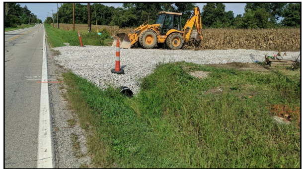
NAPD Morse Road Booster Station
