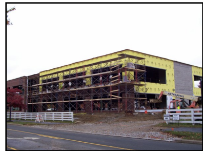
Walton Offices II
