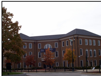
Town Center Apartments
