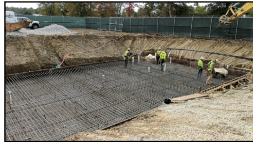
Morse Road Booster Station
