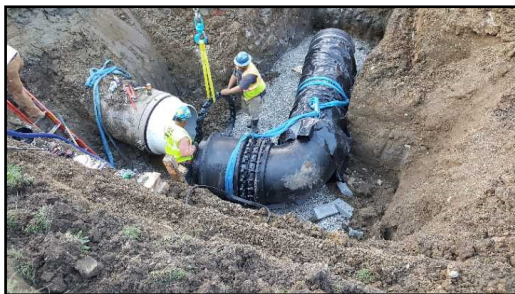
Morse Road 36in. Water Transmission Main
