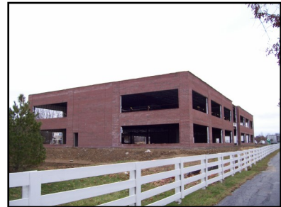
Walton Offices II
