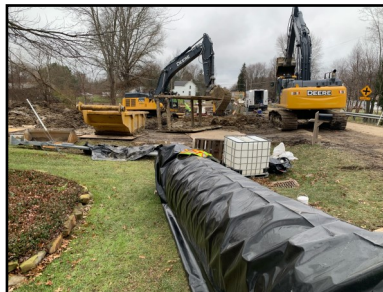
Morse Road 36in. Water Transmission Main
