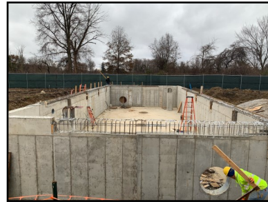
Morse Road Booster Station
