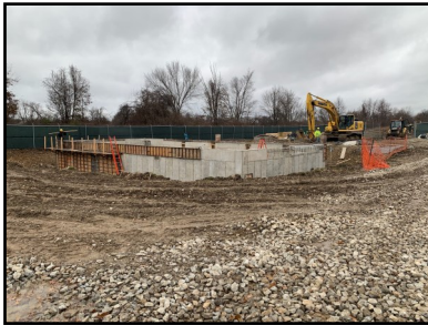
Morse Road Booster Station
