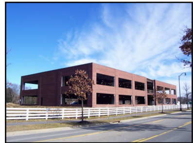
Walton Offices II
