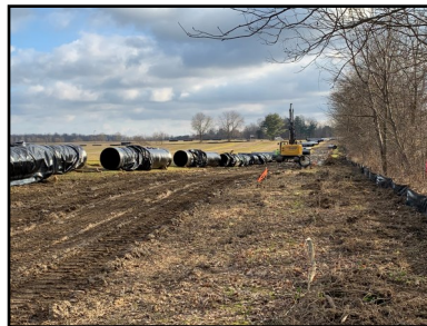
Morse Road 36in. Water Transmission Main
