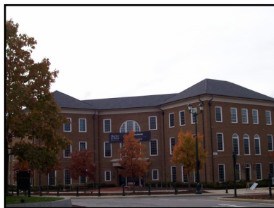
Town Center Apartments
