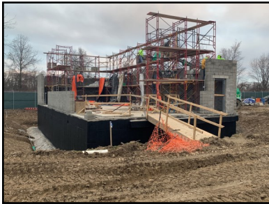
Morse Road Booster Station
