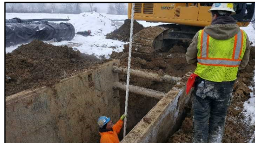
Morse Road 36in. Water Transmission Main
