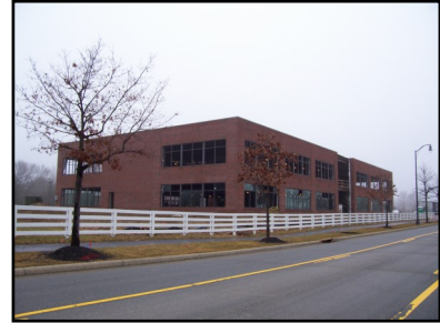
Walton Offices II
