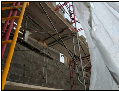
Morse Road Booster Station
