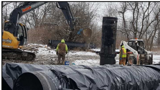
Morse Road 36in. Water Transmission Main
