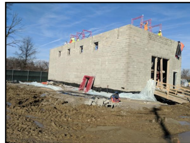
Morse Road Booster Station
