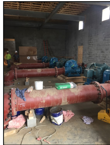
Morse Road Booster Station
