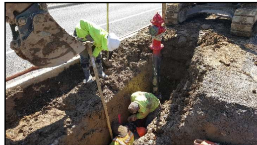
Morse Road 36in. Water Transmission Main
