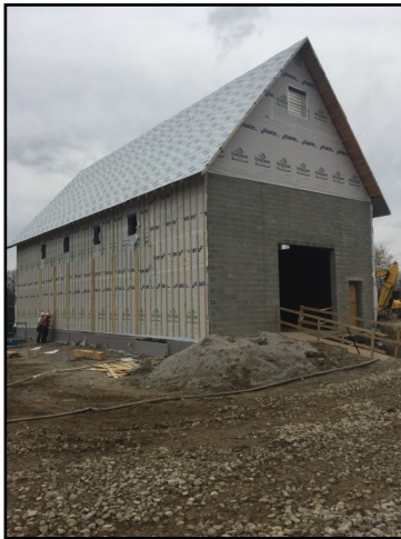
Morse Road Booster Station
