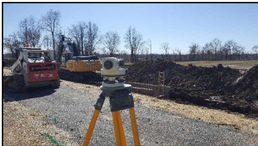
Morse Road 36in. Water Transmission Main
