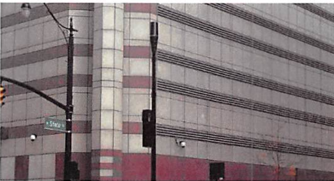
Example of a new small cell facility on a new wireless support structure.
