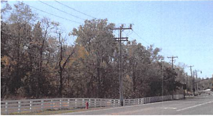
Example of an existing utility pole in the City of New Albany.
