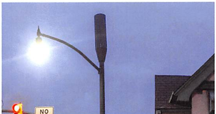
Example of top-mounted antenna on a decorative mast arm.
