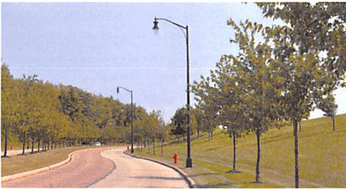
Example of existing esplanade commercial street light in the City of New Albany
