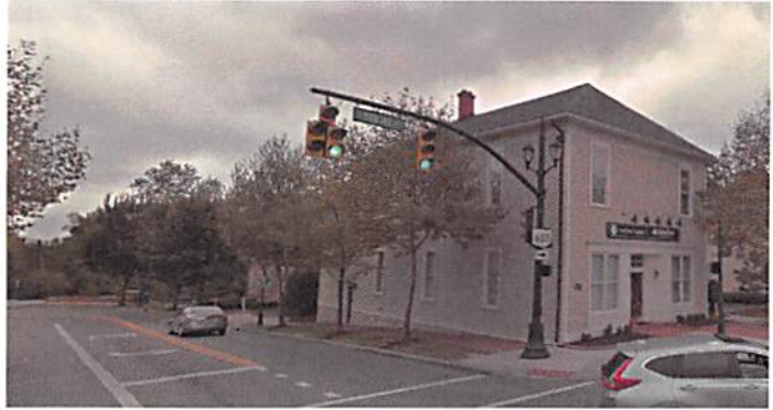
Example of existing Village Center signal mast arm.
