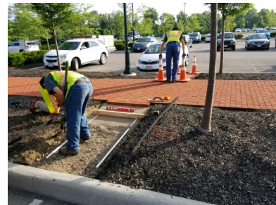
Brick pavers are placed for walkway paths at the Phil Heit Center parking lot.
