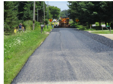
Contractors are motorpaving cold asphalt mix on Jug Street.
