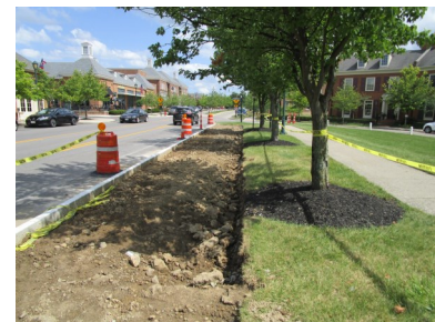
On-street parking at Market St. & Keswick Commons is removed to improve visibility.
