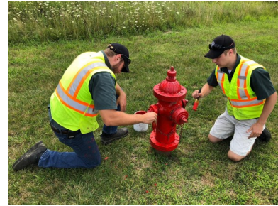
Crew members painting fire hydrant "Safety Red."
