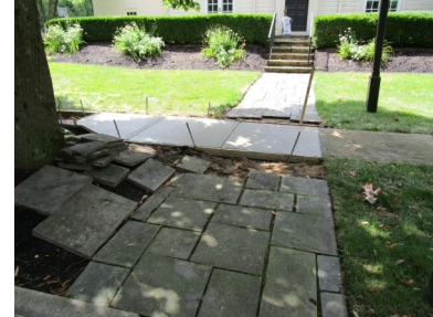
Sidewalk replacement work begins in Upper Fenway .
