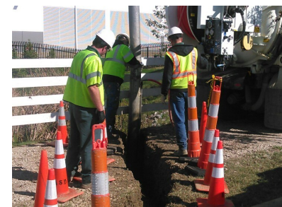
Crew members dig deep to install a storm sewer to alleviate roadway flooding.
