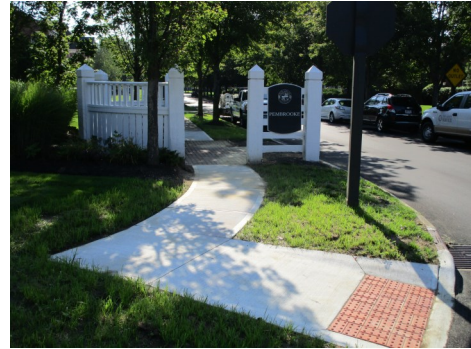
New ADA curb ramps were constructed at Pembroke Pass and Lambton Park Rd.
