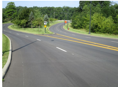
A view looking west on Smith's Mill Road after microsurfacing work was performed.
