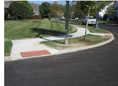
The sidewalk project included replacement ADA Ramps.
