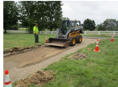
Crews construct an access ramp to the leisure trail on Brandon Road.
