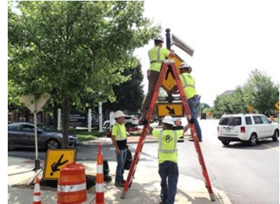
New crosswalk signals are installed and tested on Market Street.
