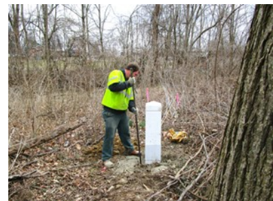
Service Worker Andrew Love installs marker posts at the New Albany Cemetery.
