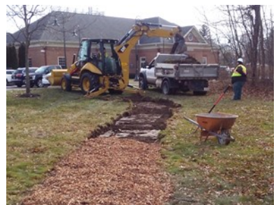
Mulch path installed between Village Hall and Police Station.
