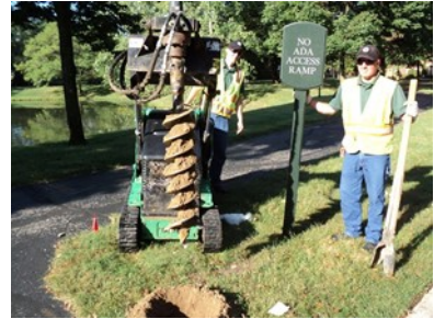
“No ADA Access” signs were placed off Olmstead Road.
