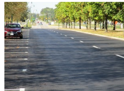
Central College Road west of SR605 was repaved.
