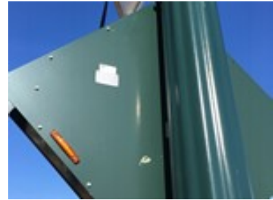
New amber indicator light on the back side of the Market/Main Ped Crossing sign.
