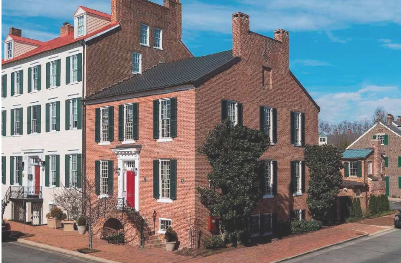
QUEEN STREET HOUSES; ALEXANDRIA, VA
