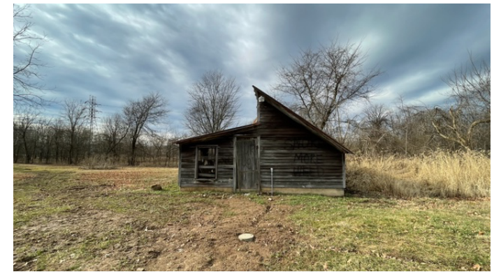
Existing Hen House
