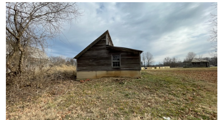
Existing Hen House
