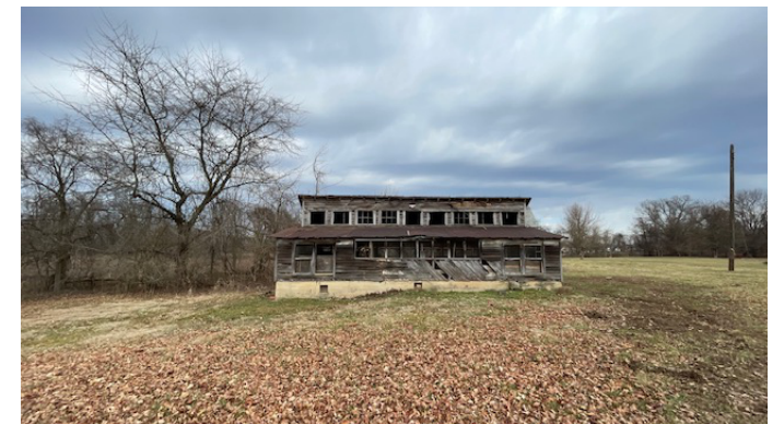
Existing Hen House
