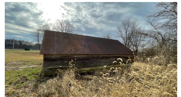
Existing Hen House
