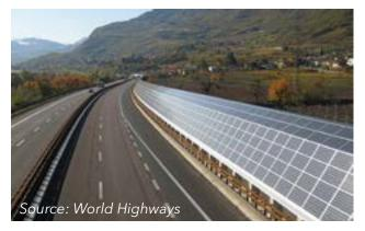
The PV barrier technique has been applied to a highway in Italy, mitigating noise pollution while generating clean energy.
