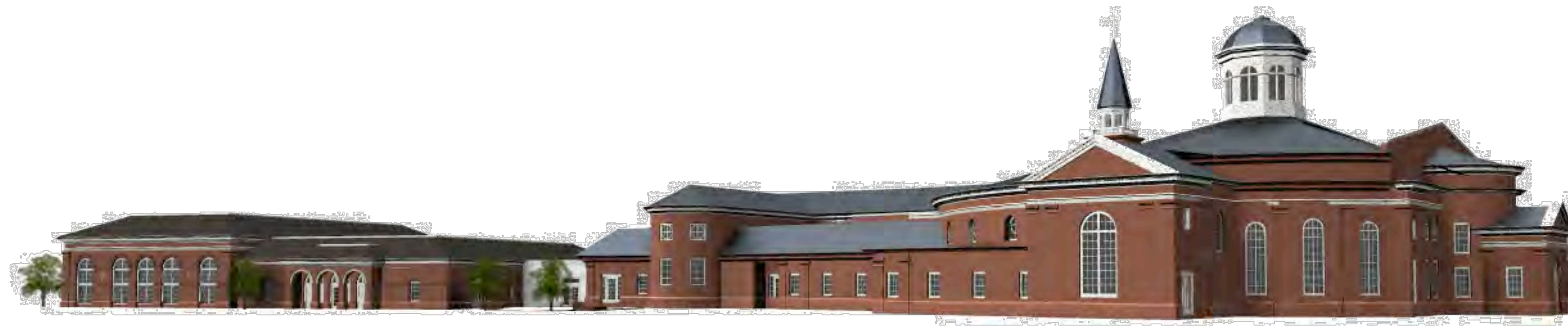
LOOKING SOUTHWEST FROM FODOR ROAD
