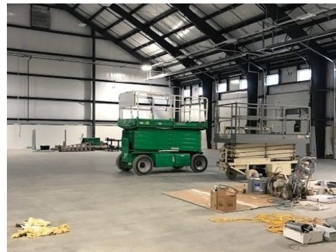
Painting contractors are organizing for their work with setting up a portable lift .
