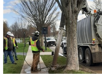
Crews hydro-excavate to access drainage pipe and remove roots.
