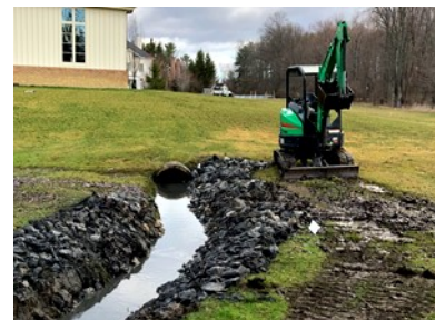
Storm ditch maintenance to improve drainage in the Waterston neighborhood.
