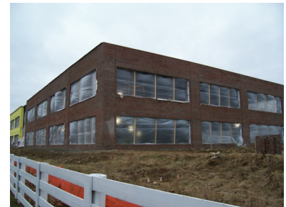
Multi-Tenant 8100 Walton Parkway
