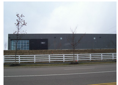
Multi-Tenant II 8820 Smith's Mill
