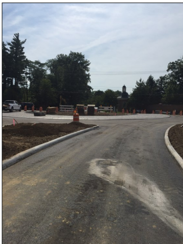
US 62/Greensward Road Roundabout looking north on US 62
