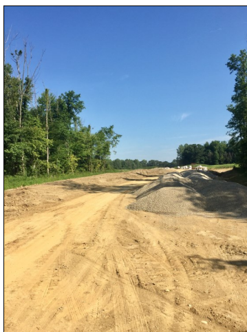
Innovation Campus Way looking west from Mink Road
