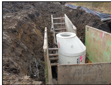
Blacklick Creek Trunk Sewer Manhole
