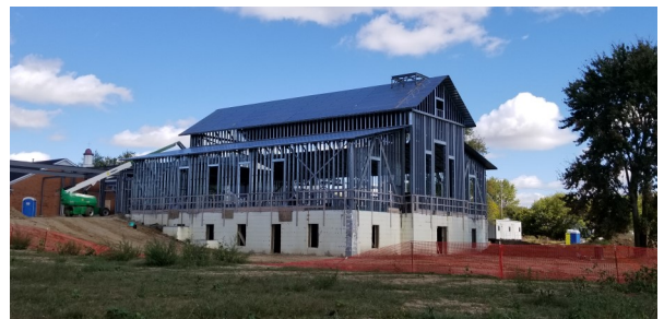
United Methodist Church Expansion
