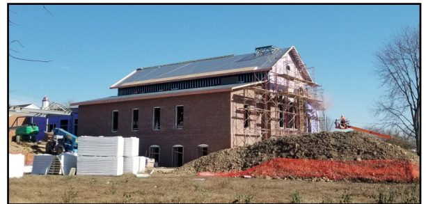
United Methodist Church Expansion
