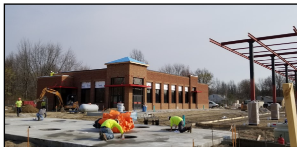
Sheetz Gas Station
