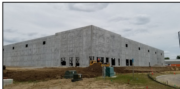
Vantrust Site J Building II
