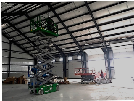
The electrical contractor is installing lighting in the new garage addition.
