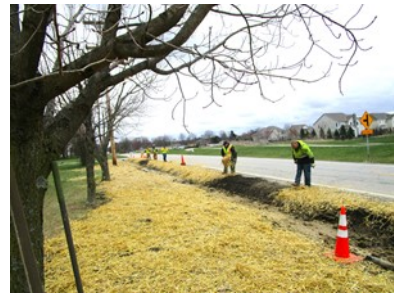
Crews place topsoil, seed and straw to complete work off Walnut Street.
