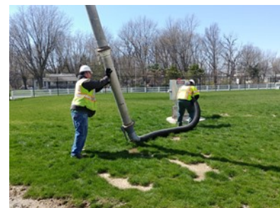
Crews clean out the sanitary lift station at the Beech Road Water Tower.
