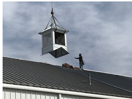
The steel erection contractor is placing the first cupola on the garage addition roof.
