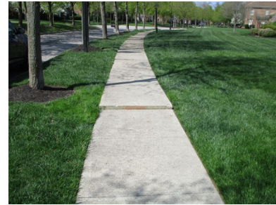
Typical sidewalk section to be replaced.
