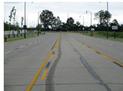
Typical roadway section designated for microsurfacing treatment.
