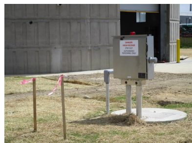
Electrical control panel for Beech Road Tank Sanitary Lift Station.
