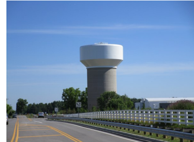
A view of the Beech Road Water Tank looking north from Beech Road.
