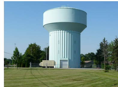
Current photo of Johnstown Road Water Tank before painting.
