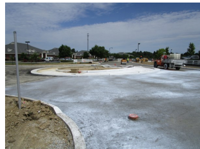
New Via Tessora Road looking north with curb and road based completed.
