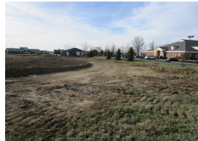
Site grading and roadway base preparation has been performed.
