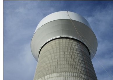
The metal tank waiting any further exterior work till April.
