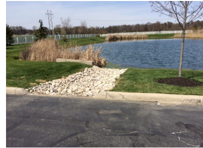
Ken Gray and Chad Bauman improve the drainage channel to the service pond.
