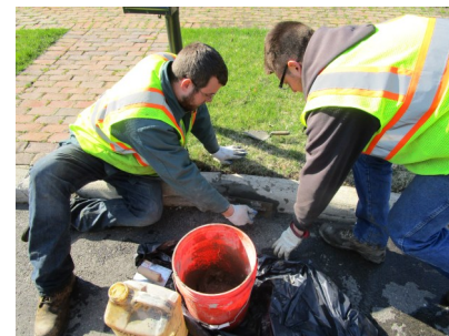
Crews patch city curb damaged by plow trucks during the winter.
