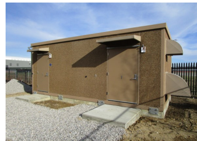
Fiber Hut building is waiting for electric and natural gas utility hook-ups.
