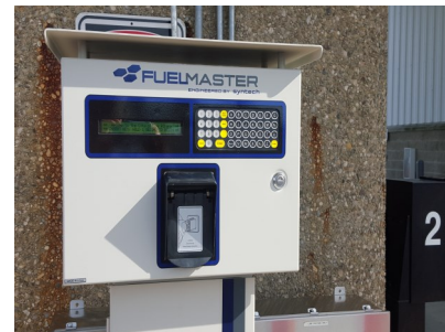
A new fuel management system is in operation at the public service facility.
