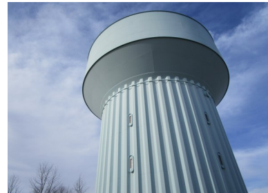
Current photo of Johnstown Road Water Tank before painting.
