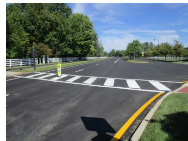
Paving on Fodor Rd. was completed and striping at the High School entrance.
