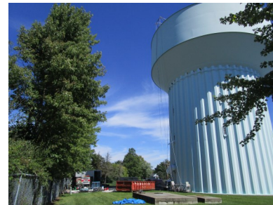
Crews are working inside the Johnstown Road Water Tank.
