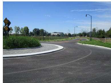
New Via Tessora Road looking at the completed traffic circle.
