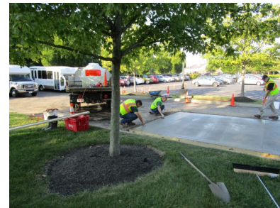
Service crew installs a new concrete pad in front of the Village Hall trash dumpster.
