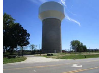
A view of the Beech Road Water Tank with the security fence installed.
