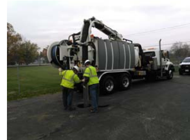
Crew members work at the Johnstown Water Tank to empty the septic tank.
