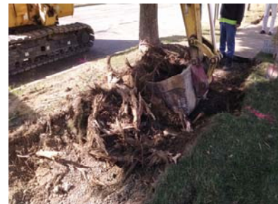
Tree roots growing beneath the concrete sidewalks have caused extensive damage.
