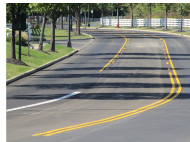
Microsurfacing was completed on Walton Parkway from SR 605 to US 62..
