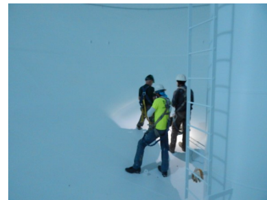
Crews are inspecting the paint applied to the inside of the tank bowl.
