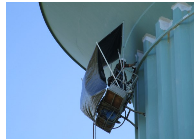
Workers painting the Johnstown Road Water Tank in September 2016.
