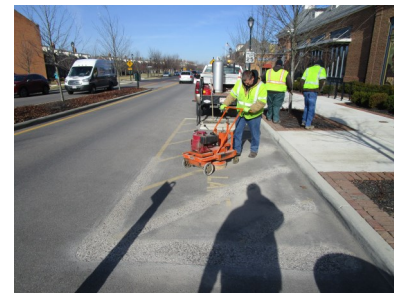
Crews install a No Parking Zone on Market Street to improve site visibility.
