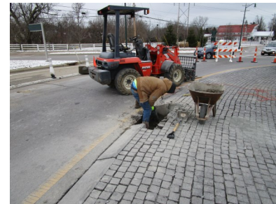
Contractors replace damaged granite curbs at the Morse & US62 roundabout.
