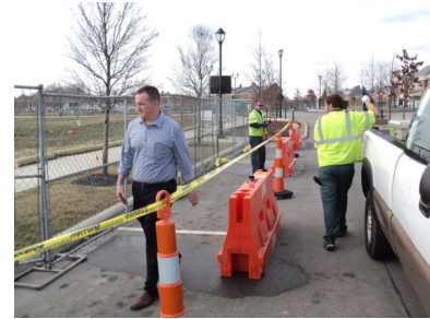
Crew members create a temporary walkway using barricades and cones.
