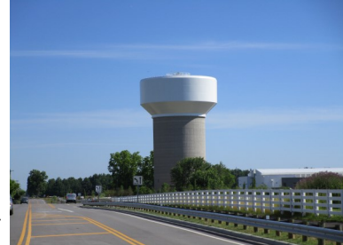
Completed Beech Road Water Tank.
