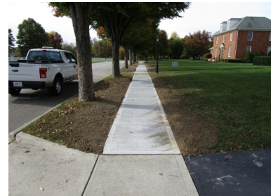
Completed sidewalks on James River Road.
