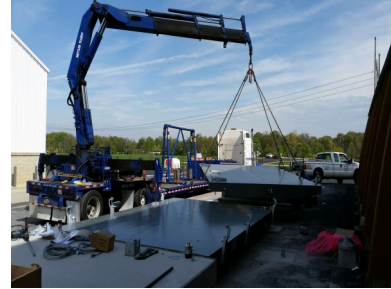
Mettler-Toledo installed a new truck scale at the public service department.
