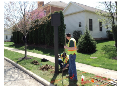
Crew members install no parking signs on Keswick Drive.
