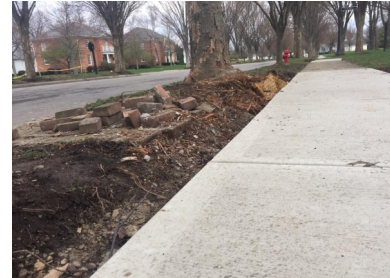
Completed sidewalks on James River Road.
