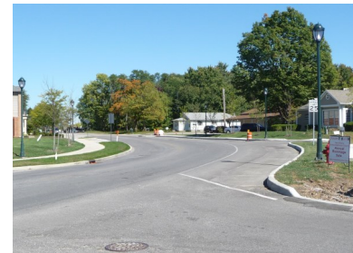
Asphalt repaving is planned for a portion of E. Main St. north of 3rd. Street
