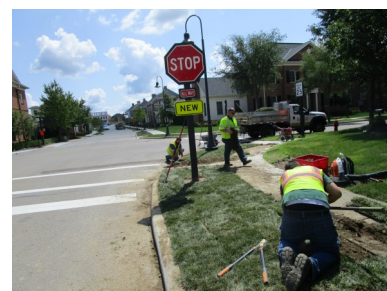
Crew members install sod to finish up ADA ramp upgrades made at Keswick & Ogden.
