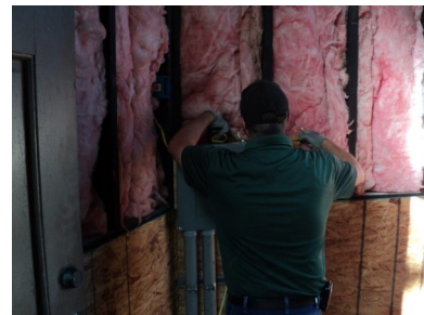
Worker Brent Rush assisted in the renovation of a new irrigation control room.
