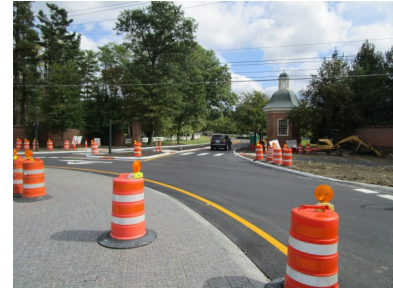
A view looking east at the partially completed roundabout center median.
