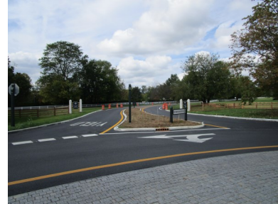
A view looking west at the roundabout connection to Greensward Road.
