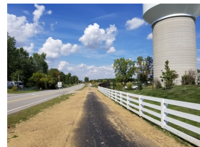
A new leisure trail was installed in front of the Beech Road Water Tower.
