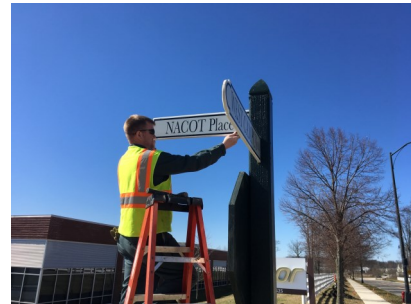
A new street name sign was installed in the business campus.
