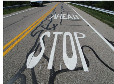
New pavement striping was performed on Kitzmiller Rd. at Dublin-Granville Rd.
