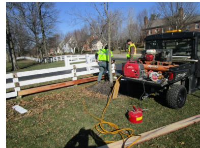
Replacement of damaged and rotten boards on James River Road.
