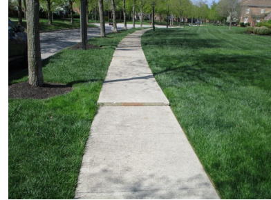
Future sidewalk replacement on Ogden Woods Boulevard
