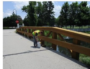
Seasonal crew member maintaining the guardrail at Hawksmoor.
