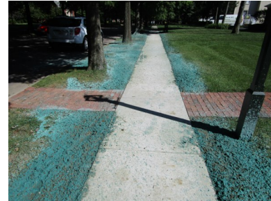
Sidewalk repair at Upper Fenway
