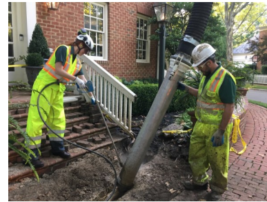
Hydro-excavating to expose and remove street tree root in Ashton Grove.
