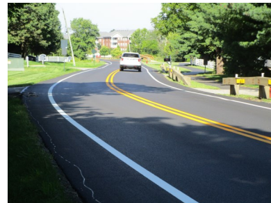
A view looking west on Thompson Road after repaving.
