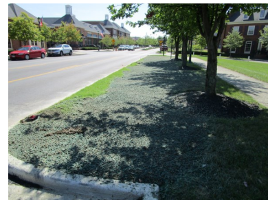
Removal of several on-street parking spaces was completed on Market Street.
