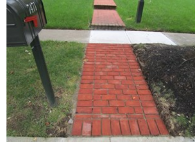
Sidewalks were replaced on Alpath Rd. eliminating trip hazards caused by roots.
