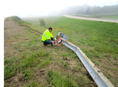
Guardrail repair is performed on State Route 161 at Beech Road.
