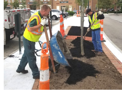
Crew members finalize the project by adding mulch to the island.
