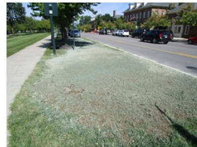
Hydro-seed and mulch was applied in September to complete the project.
