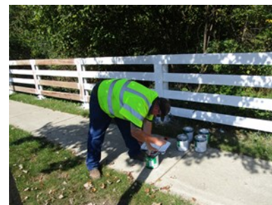
Crews repaint wood fencing along Fodor Rd. and Swickard Woods Blvd.
