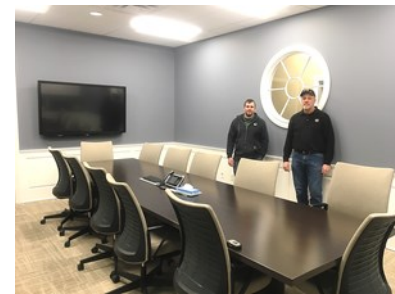
Second Floor Administration Conference Room Renovations.
