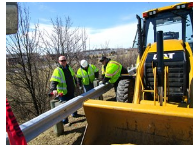
Guardrail repair is performed on State Route 161 over US 62.
