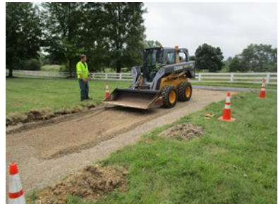
Access ramp construction to the leisure trail on Brandon Road.
