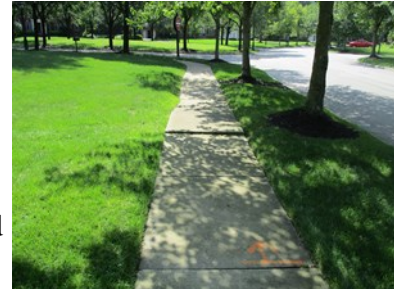
Typical sidewalk section to be replaced.
