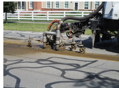
Removal of striping for application of microsurfacing on Dublin-Granville Rd.
