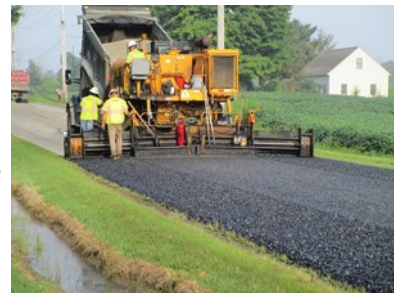
Motor grading paving on Jug Street between Beech and Harrison Road.
