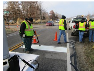
New stop bars for an All-Way Stop are installed.
