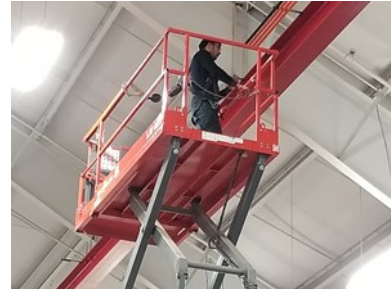
Behob Corporation installs a new motorized crane.
